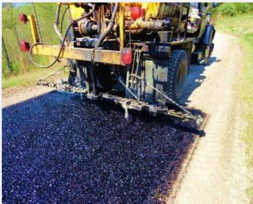
Application of Conventional-Asphalt Chip Seal in Whitley County, 2016 Photo by Christopher “Kitt” Tuttle
